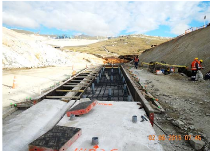
Figure 18-39: Forming the grout curtain and the PVC composite membrane anchorage on the exposed dam abutments
