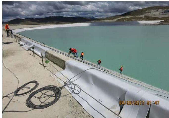
Figure 18-40: Installation of the PVC membrane over the porous concrete facing
