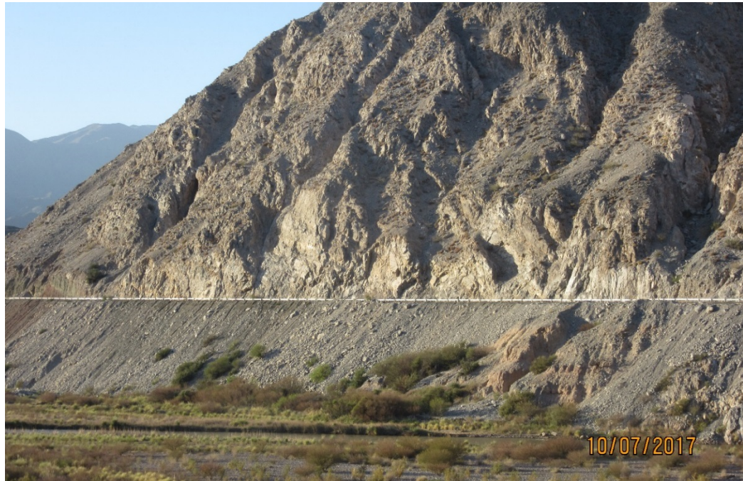
Figure 26-3 A road constructed through the challenging section of the Northern Route would look similar to this road excavated in a very steep rock slope with the road platform well above any potential peak river flow.
