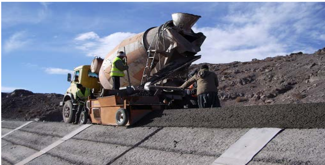
Figure 18-32: Typical Construction of the slip-cast porous concrete section which anchors the strips of lining material used for fixing the composite liner.
