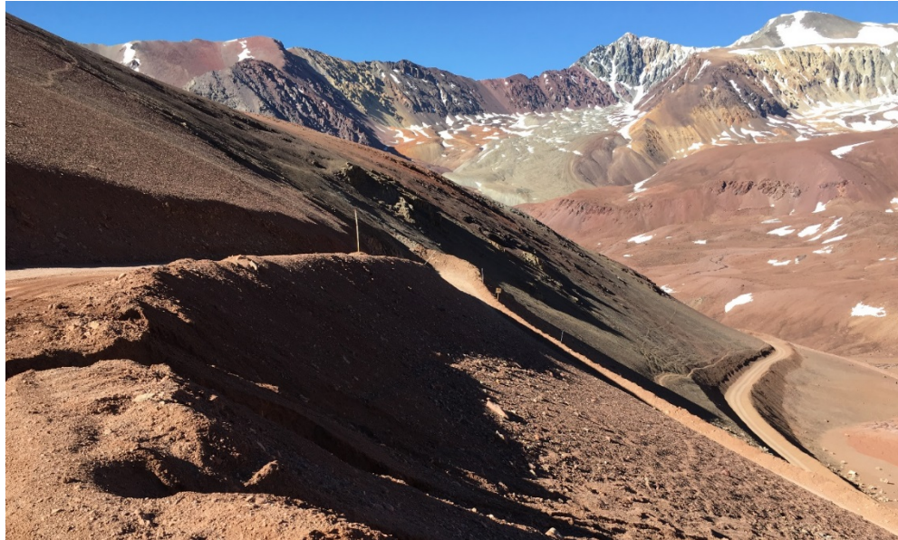
Figure 18-2: Recently graded hair pin bends during January 2017 at Totorá Pass on the existing central route to Los Azules, elevation ~4,200 masl.
