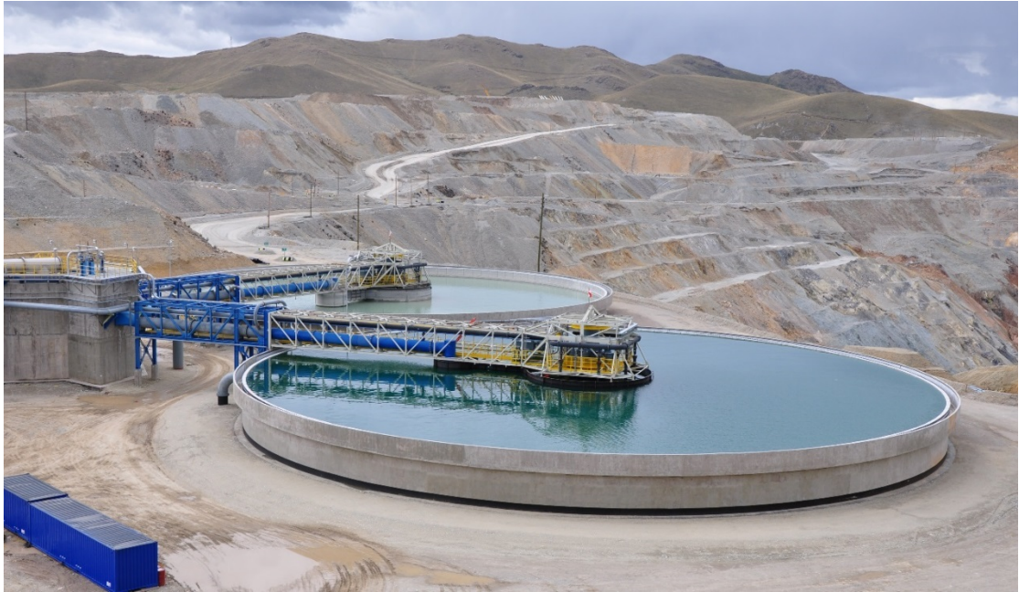
Figure 17-9: Antapaccay Tailings Thickeners
