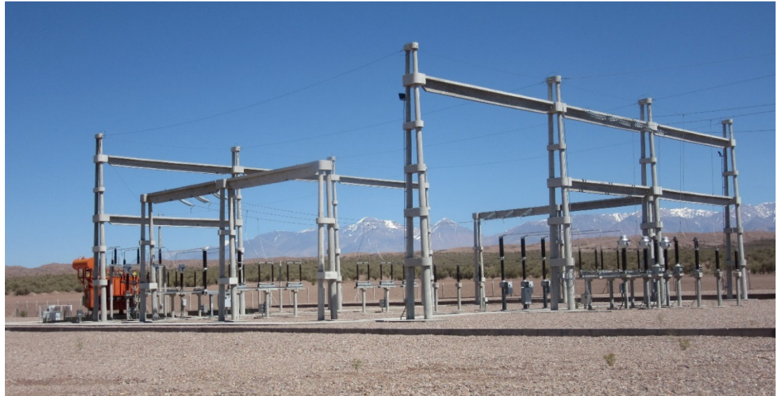
Figure 26-5 The new substation yard at Calingasta, presently occupied by a single orange transformer feeding the local township.
