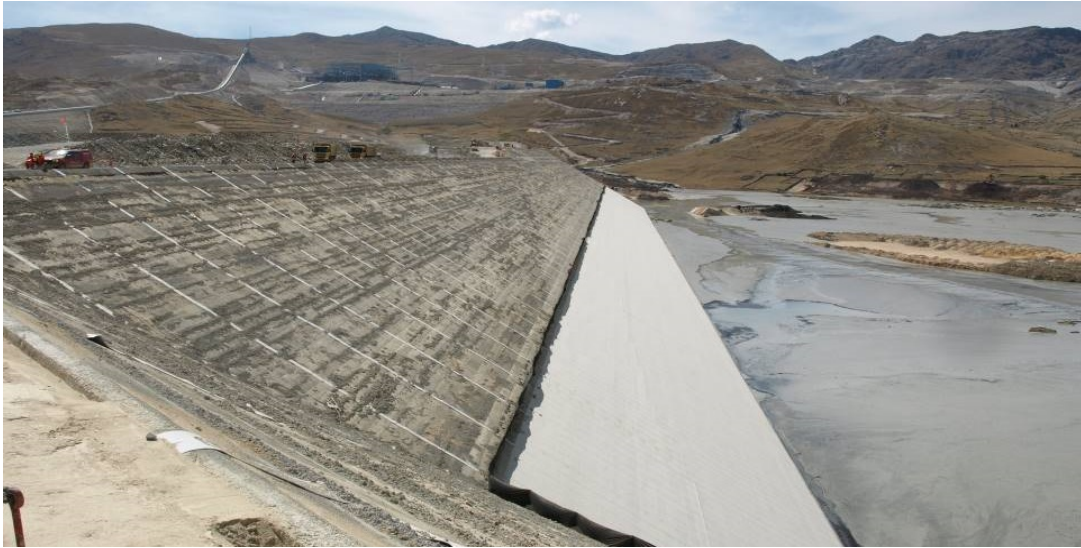
Figure 18-33: Staged construction of upstream face with slip-formed concrete base, and partially placed geocomposite liner.
