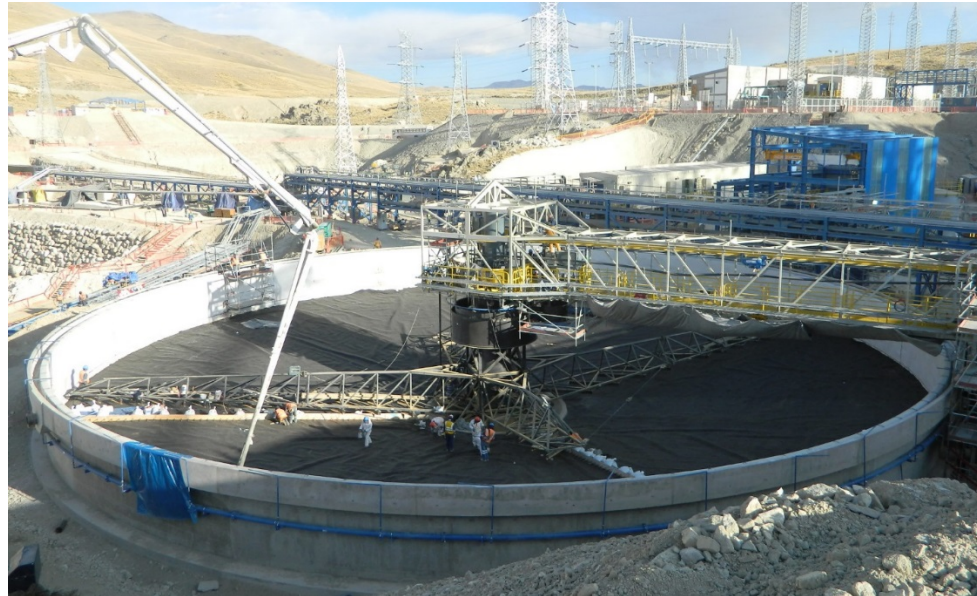
Figure 17-21: Concentrate Thickener Under Construction
