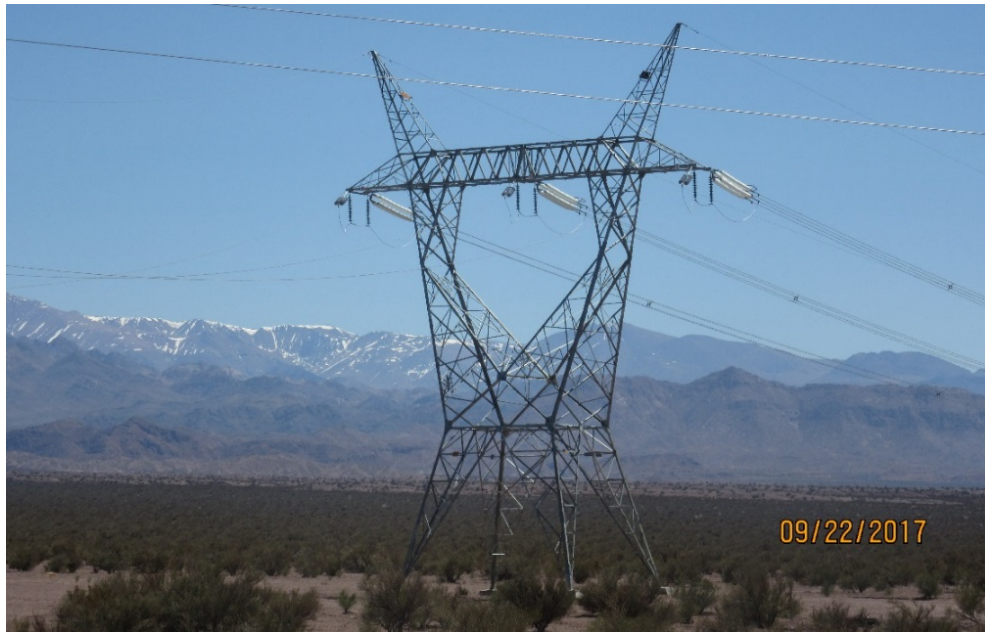
Figure 26-4 The 500kV transmission line final tower at Calingasta constructed in anticipation of large mining projects in the high Andes. Presently energised at 128kV for the small population of Calingasta.
